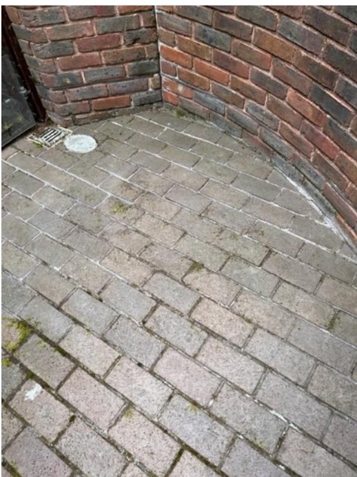
3 After treatment with Weed Ripper
